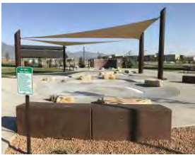
Integral Color Concrete Seat Wall
